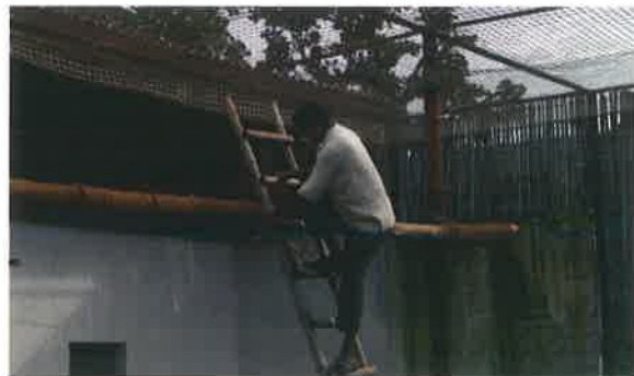
Repair of perches
