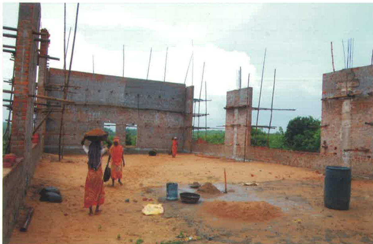
Colony aviary under construction
