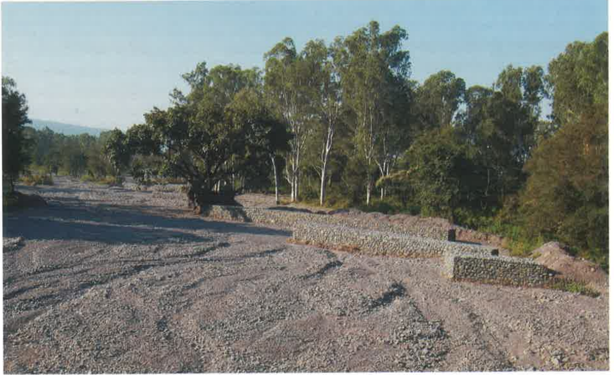
Spurs on the river bed prevent inflow of water to the Centre during floods
