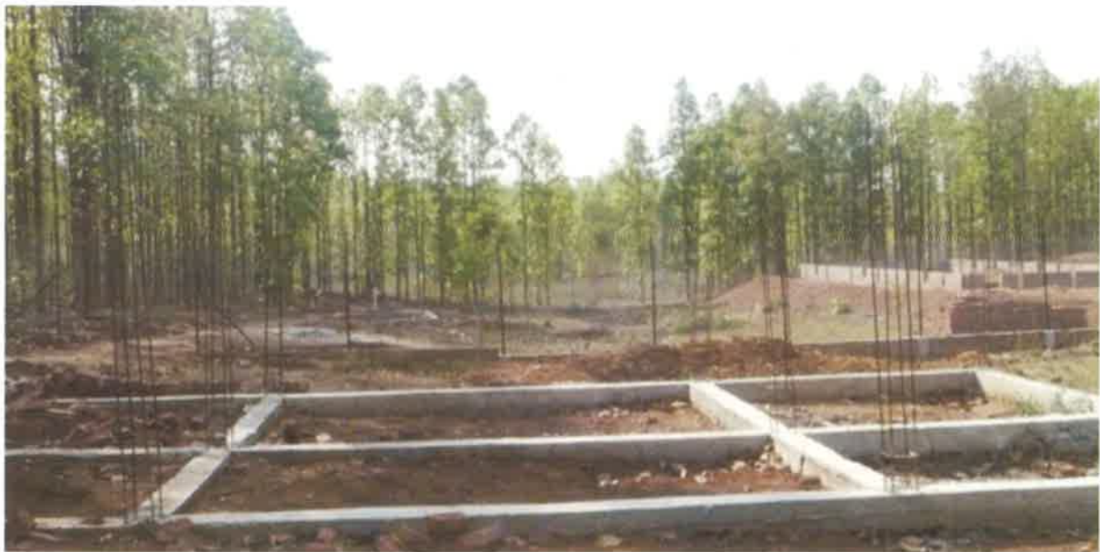
Office building under construction
