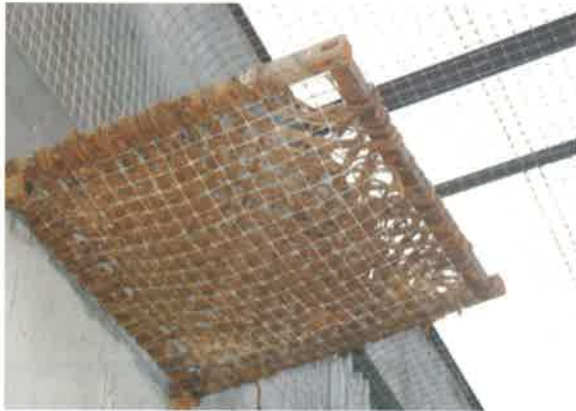
Newly installed wooden cot in the aviary
