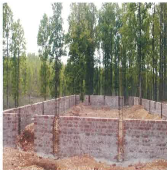
Colony aviary under construction
