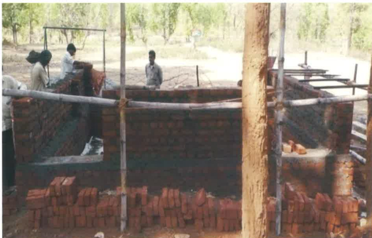
Quarantine pen under construction
