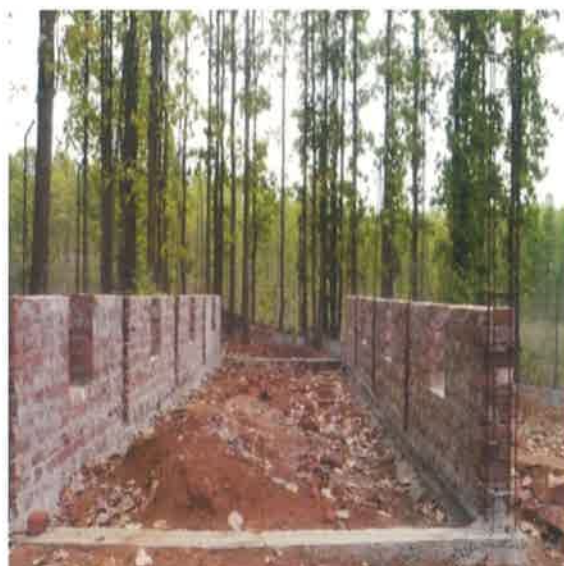
Nursery aviary under construction
